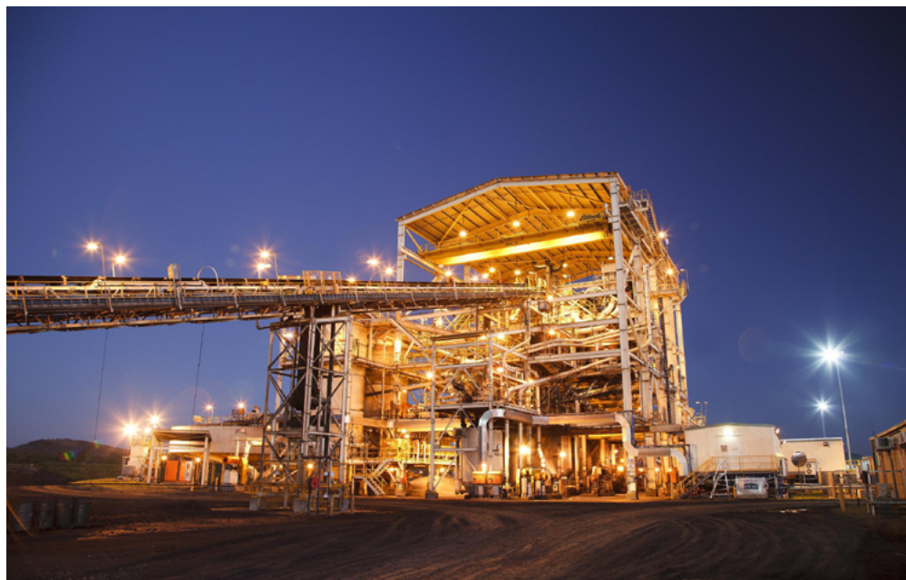
The wash plant at Sonoma Mine
